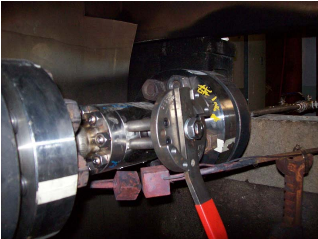
Valve Prior to Test
