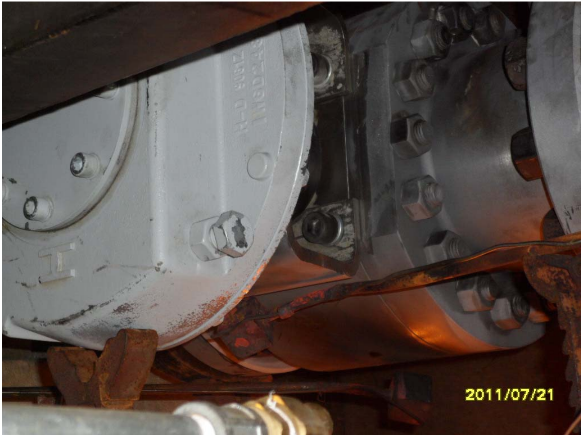
Valve Prior to Test
