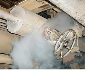
*Globe type valves often develop dangerous leak paths due to their torque seated design. Their linear operation requires an operator to seat the plug by exterior force, often repetitively as the flow stream can cause the valve to become unseated.*
