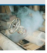
Leaking valves are costing power plants millions in lost energy and maintenance down-time.
