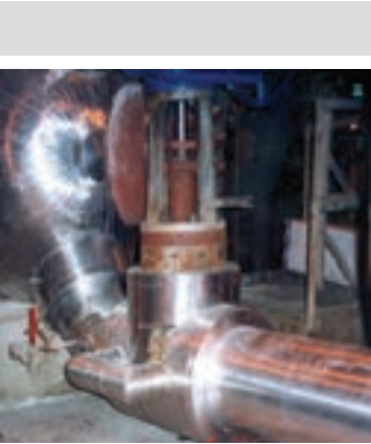
Pictured above is an ASME / ANSI Class 2500 Parallel Slide Gate Valve (PSGV) installed in a high pressure feedwater isolation application. If the heater has a tube leak, it must be isolated for repair. On units with elevated pressures, the PSGV allows for repeated leak free isolation.
