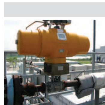
This ValvTechnologies' valve is installed in a cogeneration facility on the Gulf Coast. The application pictured is a vent valve located in the reheater section of the HRSG.
