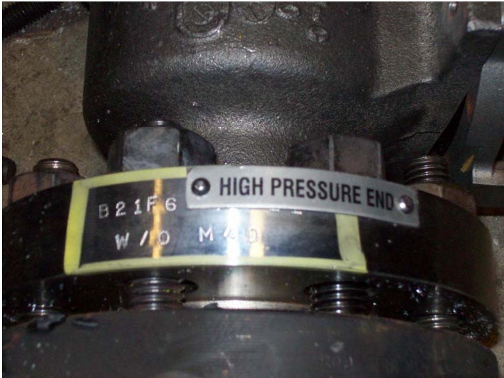
Test Valve Before Test
