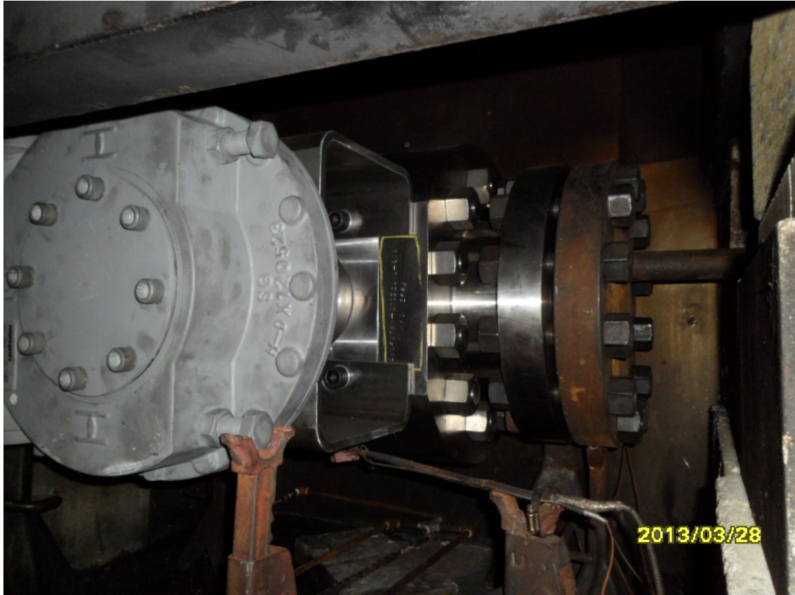
Test Valve Setup Prior to Burn
