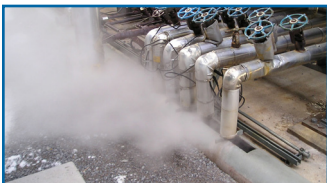
Leaking valves
