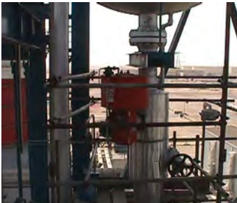
Pictured above: This Electronic Relief Valve (ERV) was installed to provide protection to the safety relief valves, which if operated could cost the plant thousands of dollars in replacement.
