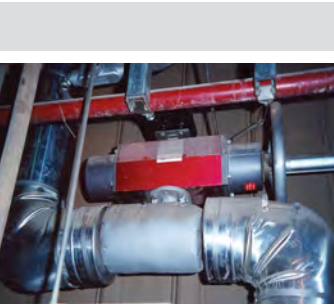
Pictured right and above are boiler feed pump recirculation valves. These ValvTechnologies' XACTROL® models have been in successful operation for over eight years without requiring trim or packing replacement.
