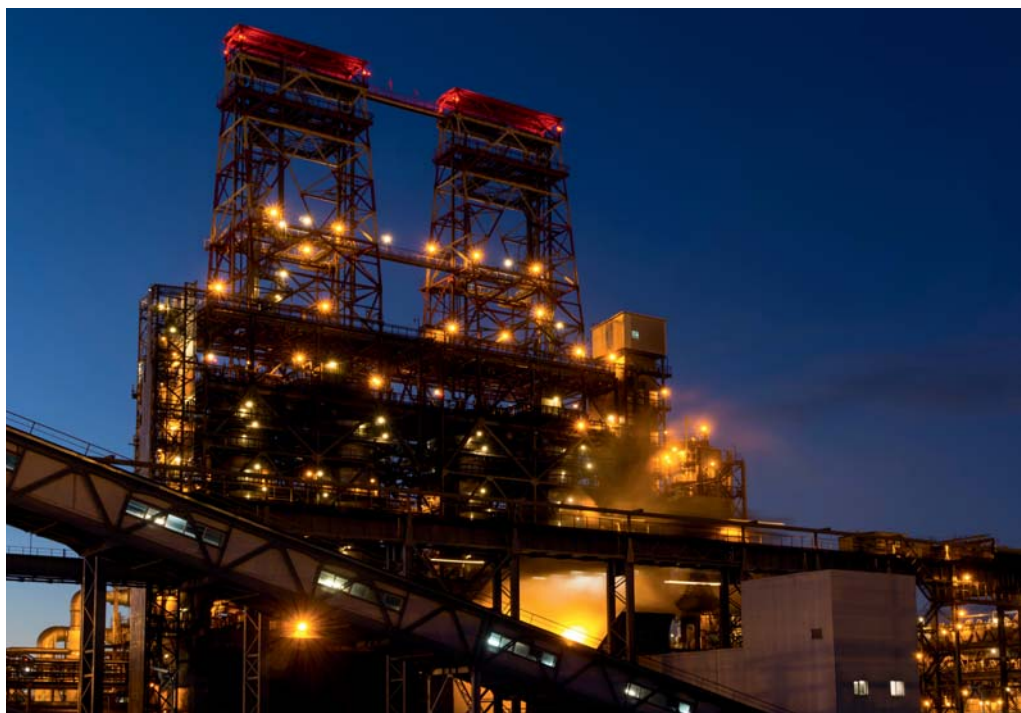
4-drum delayed coking unit in a petroleum refinery
