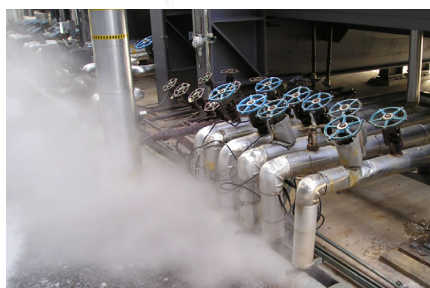
Leaking valves
