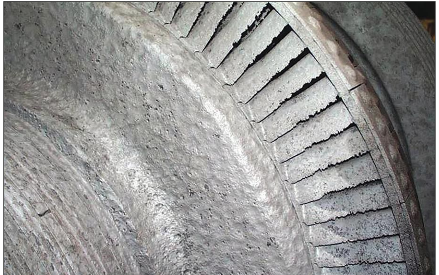
Figure 2. HP turbine first-stage damage due to liberated pieces of hardfacing.
