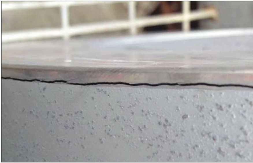
Figure 3. Interfacial crack at base metal substrate and hardface boundary.
