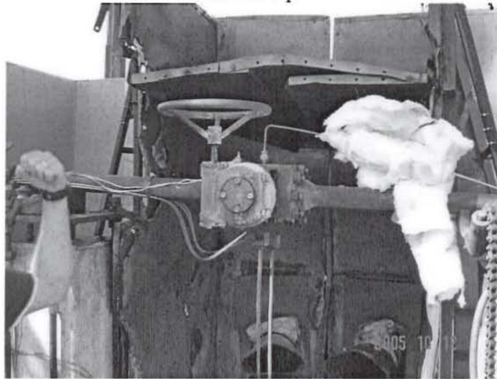
Valve after completion of Burn
